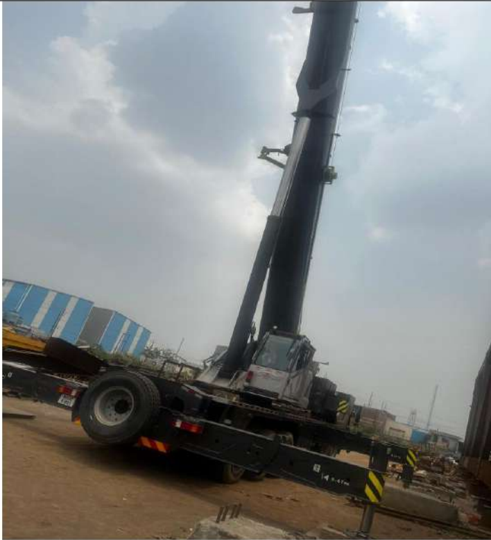
150 MT MOBILE CRANE
