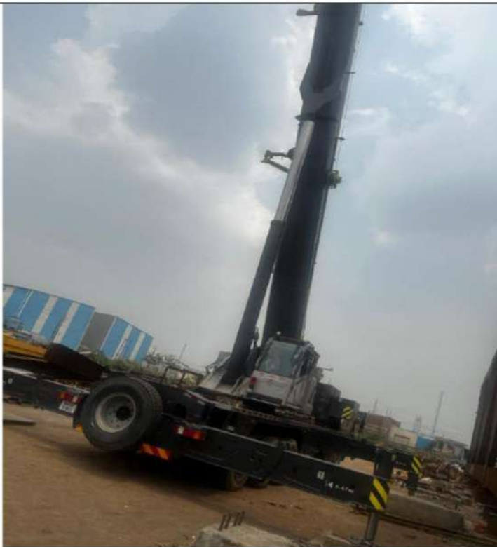
150 MT MOBILE CRANE
