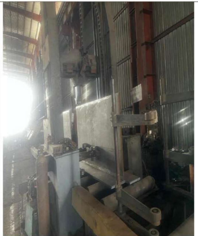
BEAM FITUP MACHINE
